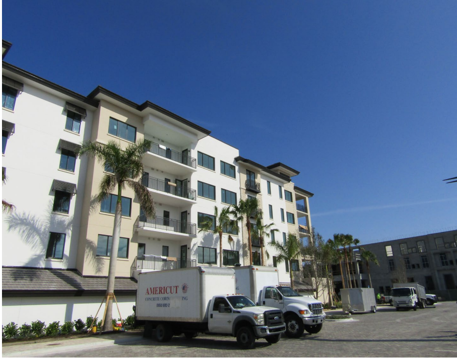
Photo 3 – Partial South elevation.
