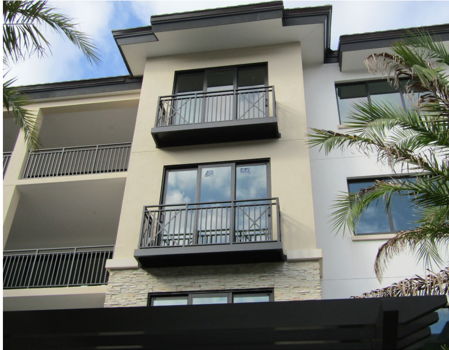
Photo 9 – View of typical pre-engineered Juliet balconies.
