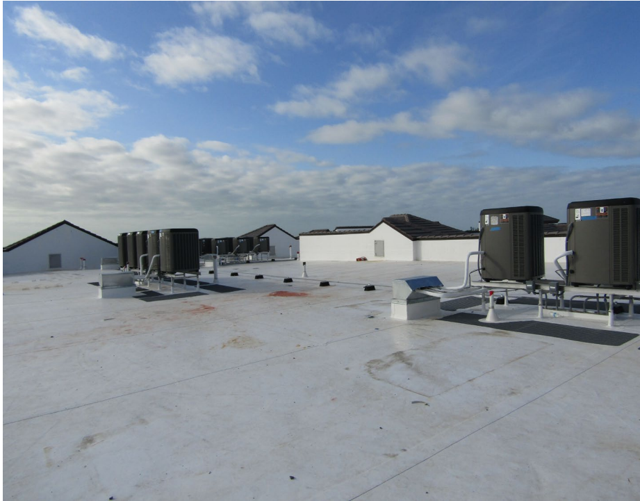
Photo 5 – Partial view of TPO roof system.
