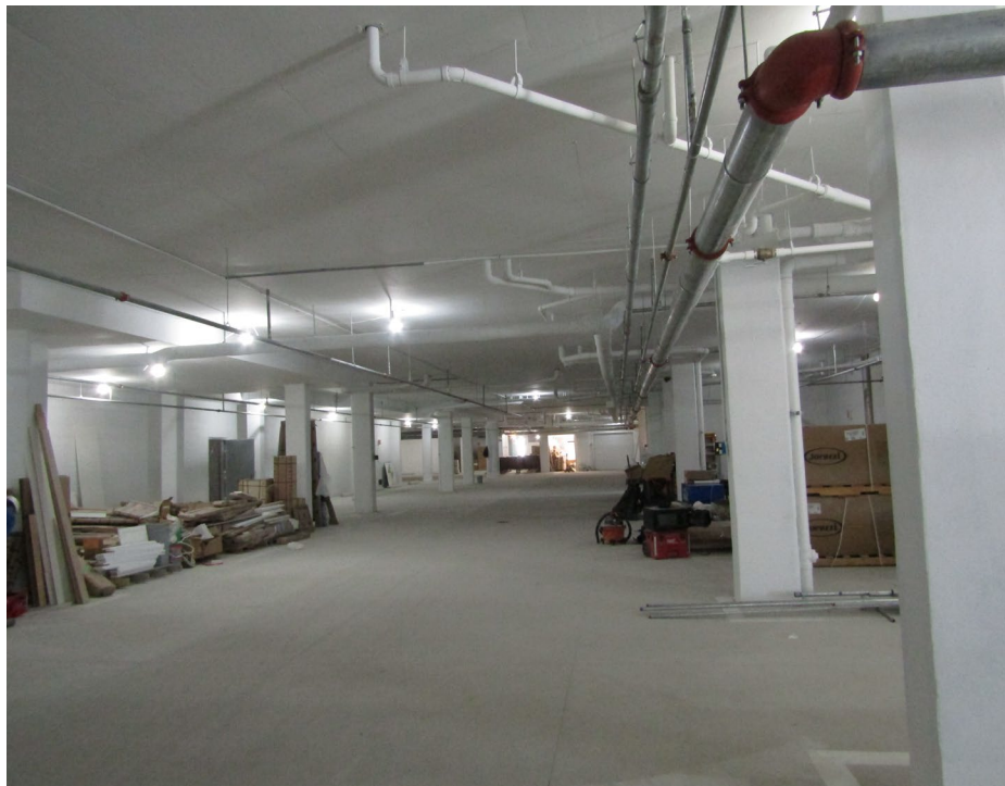
Photo 10 – Partial view of Parking garage.
