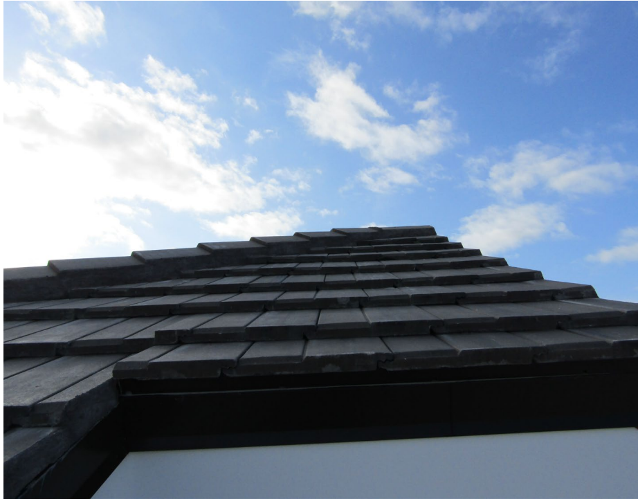
Photo 7 – View of typical concrete tile hip roof system.
